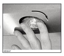
11.2 Install trim rings by pushing upward.
